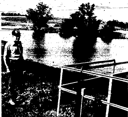
GRADED STRUCTURE, which takes the place of a road bridge gets inspection by commissioner Floyd Burt.
